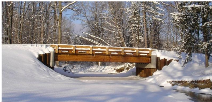
Bennington Bridge No. 4 (under $1M)
